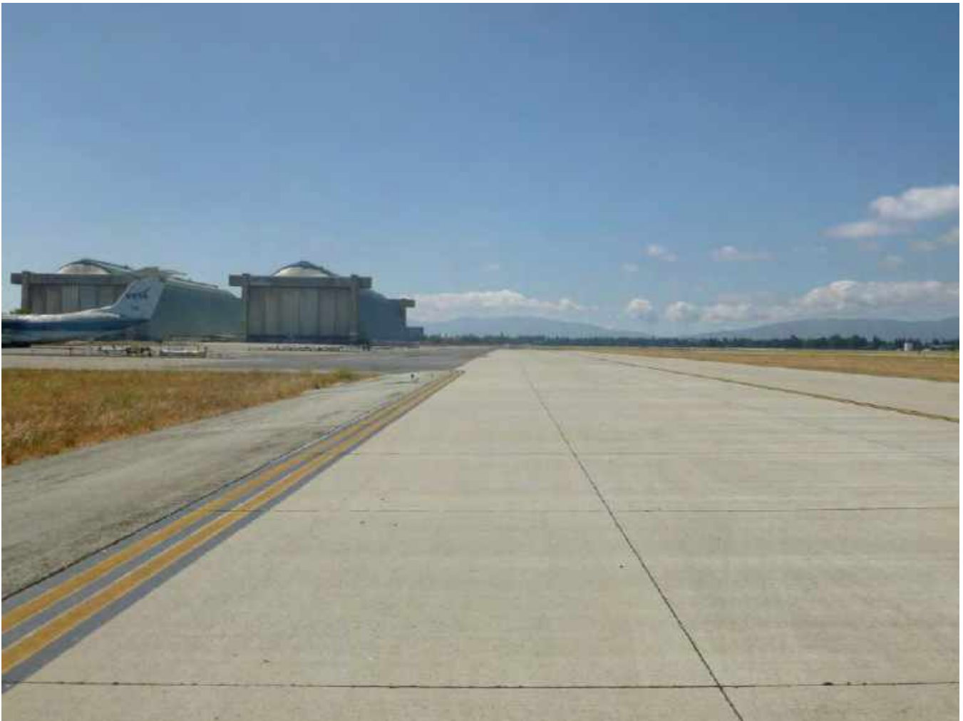
View of east parallel taxiway looking south toward Hangars 2 and 3 (Source: AECOM 2013)
