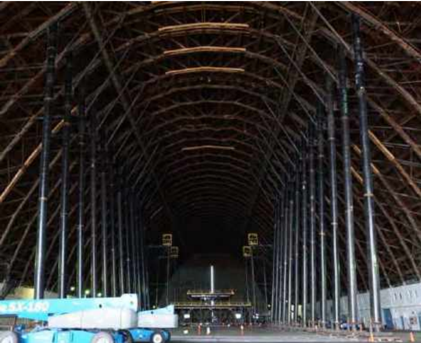
Temporary shores after installation
