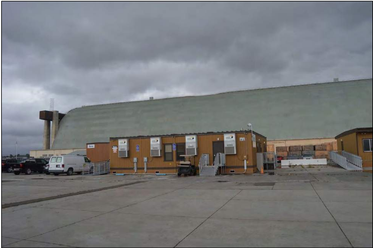
Photograph 1: East elevation of Hangar 3, looking southwest. Note the dip in the roofline at center, indicating the partial roof failure.
