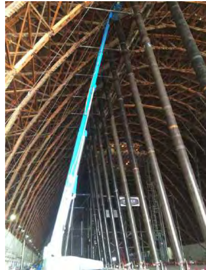
Boom lift used for visual observations
