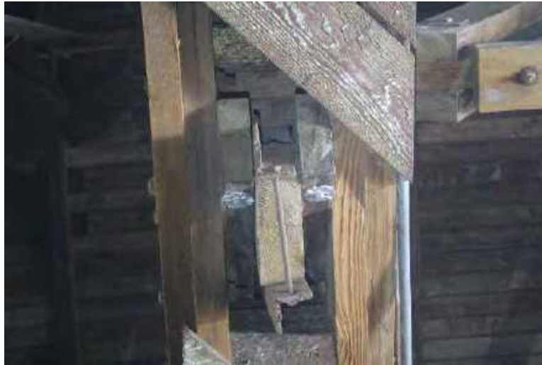
Figure 17. Example of new minor connection strengthening stitch bolts adjacent to existing angle clamp.
