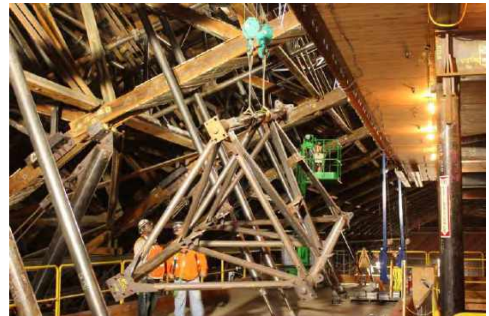
Hoisting exoskeleton segment into place
