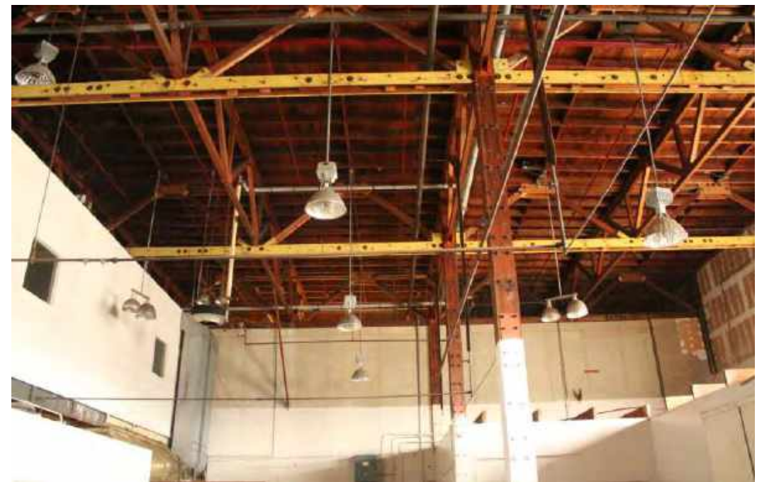
Interior view of Hangar 3 East Shed Annex
