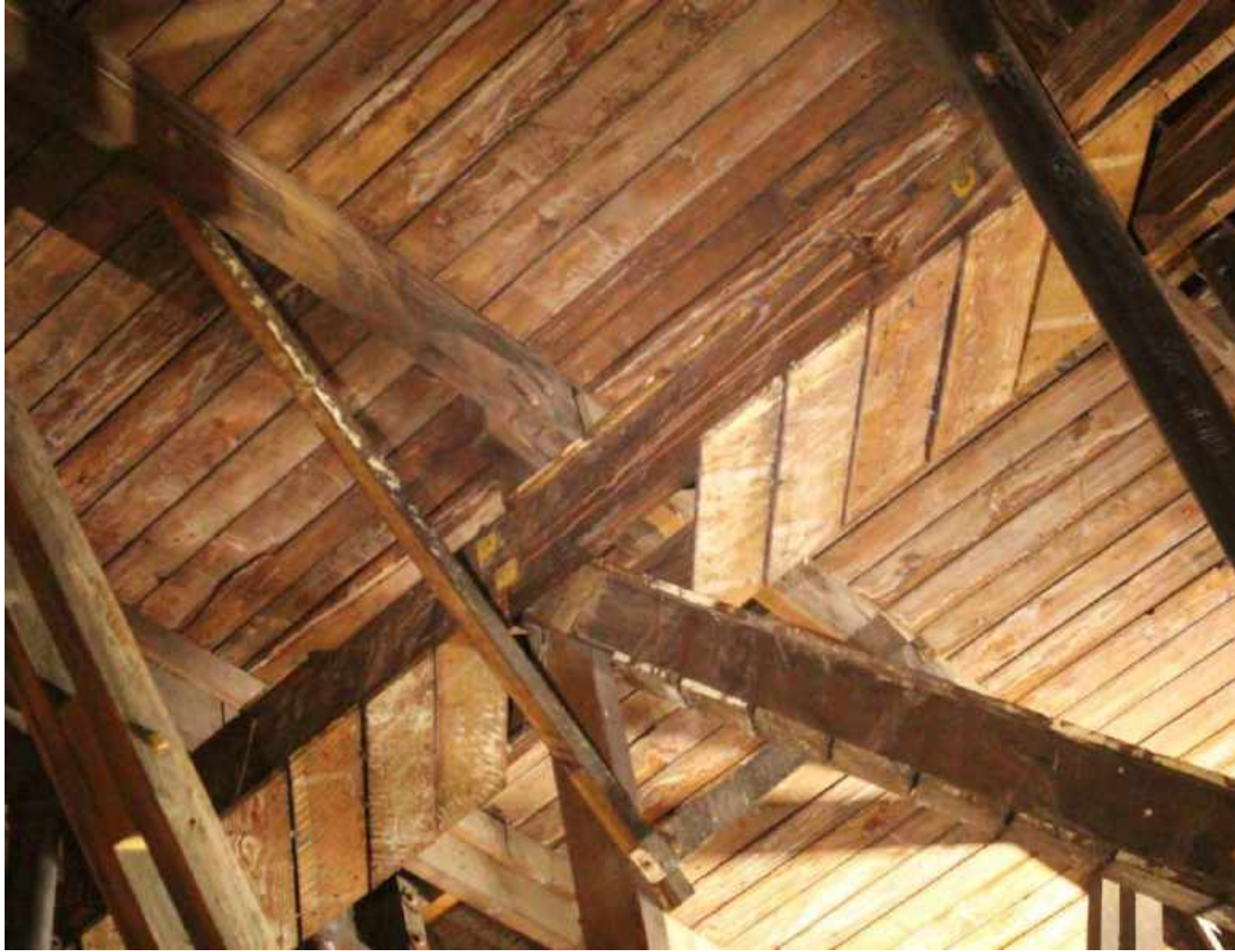
Typical vertical web member with added knee-braces
